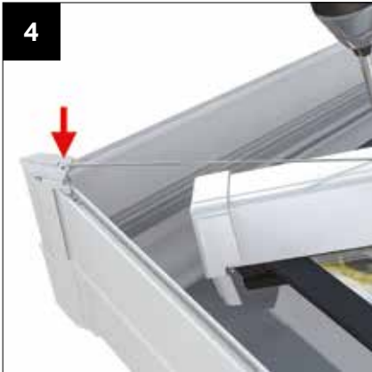
4 Finally, fix the tie wire using CRN010 screws, to secure the corner.
