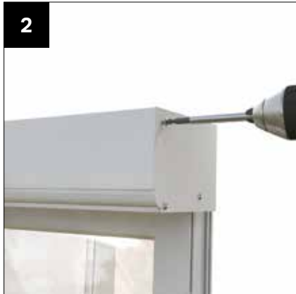
GUTTER STOP END DETAIL - Used with lean-to roofs, gable roofs or when then gutter returns along the host wall. Secure the end plate into position using the fixings provided (CRN008).
