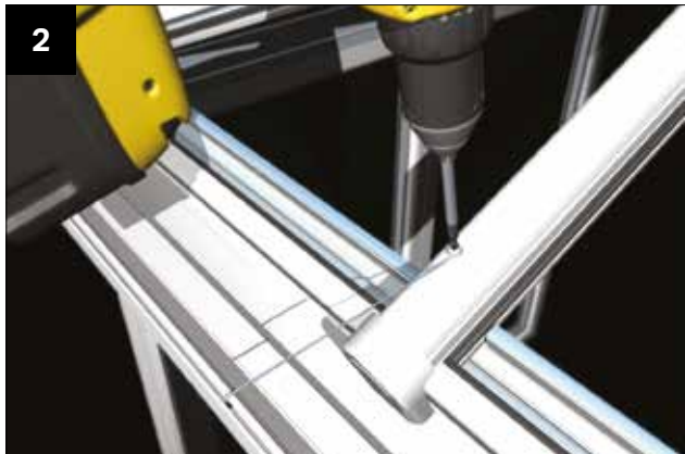
2 Secure the upper Cornice section using the wire ties at each glazing bar. Hook the wire tie into the pre-drilled hole in the upper Cornice section and screw fix into the glazing bar, ensuring the upper section remains parallel to the frames/roof line.
