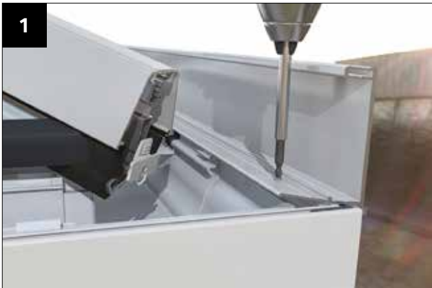
1 Temporarily support and fit the upper Cornice section, using the fixings provided (FSD-42-19).
