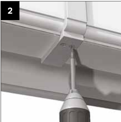
2 Whilst ensuring that the corner remains located in position, screw fix using self drilling screws CRN007
