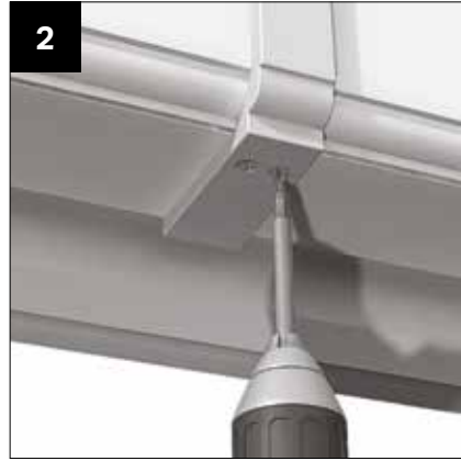
Whilst ensuring that the corner remains located in position, screw fix using self drilling screws CRN007.
